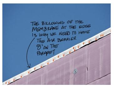
The peel and stick joints (typically rubberized asphalt) is not compatible with roof membranes.
